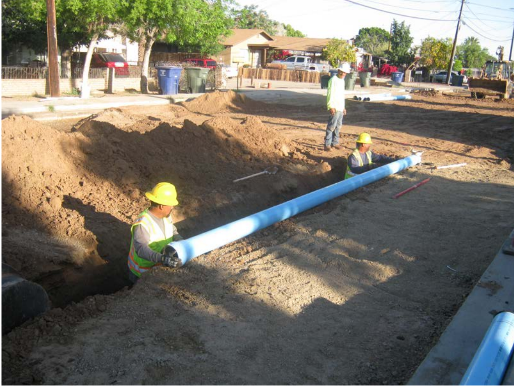
Figure 6. Closure of entire street for open-cut
