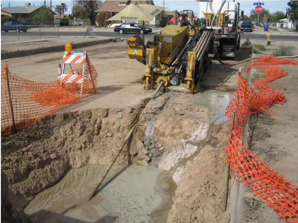
Figure 7. Partial street closure for HDD installation
